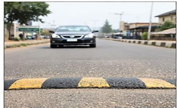
Figure 2. Speed Bump on Odota-Airport Road
