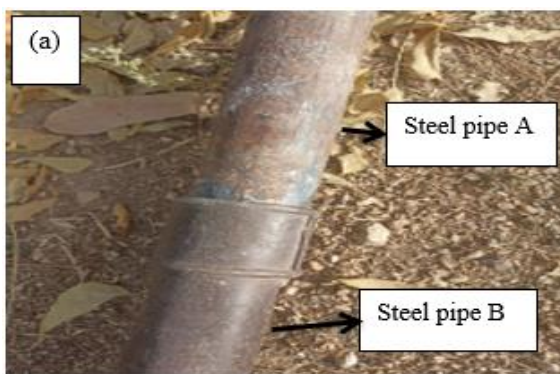
Fig. 1: Steel pipes from a borehole site (a) Couple steel pipes removed from a borehole
